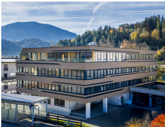
© Schian.at | Holzbau Saurer
